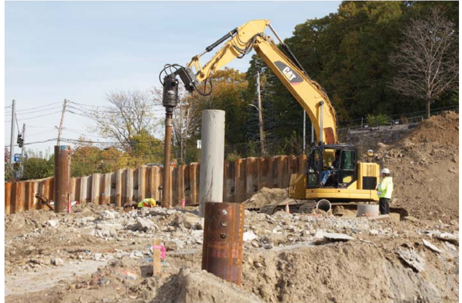
8.625" HELICAL PIPE PILES GREATLY IMPROVED PRODUCTION TIME, RESULTING IN SIGNIFICANT COST SAVINGS.
