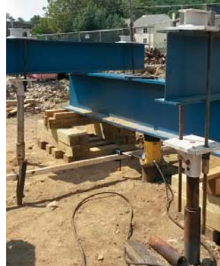
8.625" HELICAL PIPE PILES GREATLY IMPROVED PRODUCTION TIME, RESULTING IN SIGNIFICANT COST SAVINGS.
