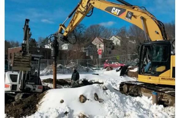
8.625" HELICAL PIPE PILES GREATLY IMPROVED PRODUCTION TIME, RESULTING IN SIGNIFICANT COST SAVINGS.
