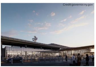
THE HEADHOUSE EXPANSION **EXTENDS UNDER THE EXISTING ELEVATED 4-LANE DEPARTURES ROADWAY AND THE PARALLEL** AIRTRAIN, BOTH OF WHICH HAD TO REMAIN OPERATIONAL **DURING INSTALLATION.**
